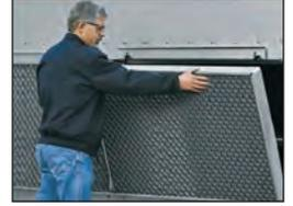
**Clean Pan:** EVAPCO units feature a completely sloped design from the upper to the lower pan section. This "Clean Pan" design allows the water to be completely drained from the basin.
